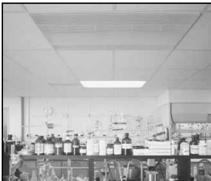
Chemistry Lab with TriTec Diffusers
